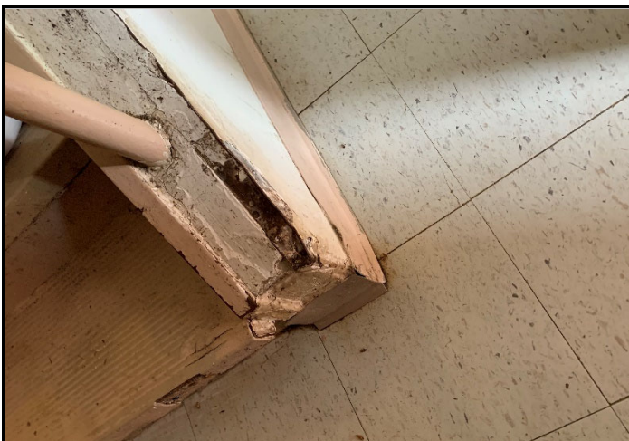
Photo 11: Typical brittle plaster conditions throughout.
