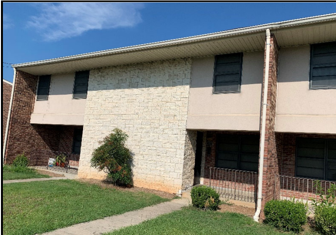
EIFS siding and sim-stone additions in 1996 faulty, but also add generic 1-dimensional look to the facades
