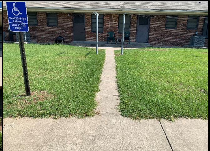
Lack of handicap accessible site design, including lack of adequate curb cuts, ramps, or sufficient sidewalk width
