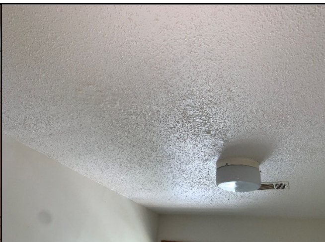
Photo 12: Example of ceiling damage due to moisture infiltration (roofing)
