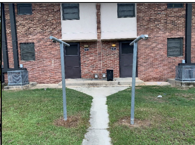
Photo 6: Example of poor sidewalks (inadequate width and drainage) and unused laundry line poles
