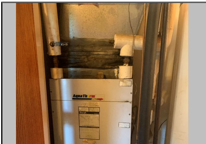
Photo 9: Aquatherm HVAC units need redesign and replacement. They do not operate well for the property.
