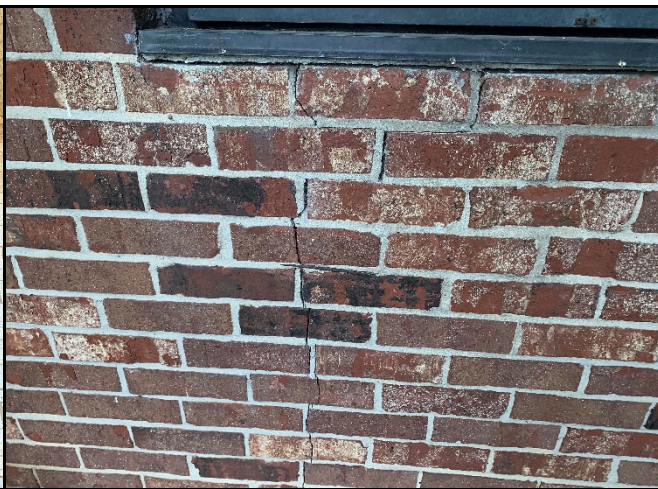
Photo 2: Typical stairstep structural cracking at brick
