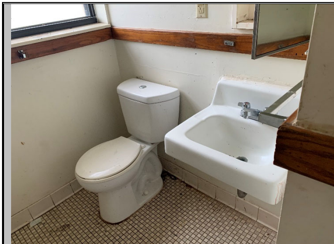
Photo 7: Original bathroom sink, fixtures and ceramic flooring (note toilet is a replaced water saving device)
