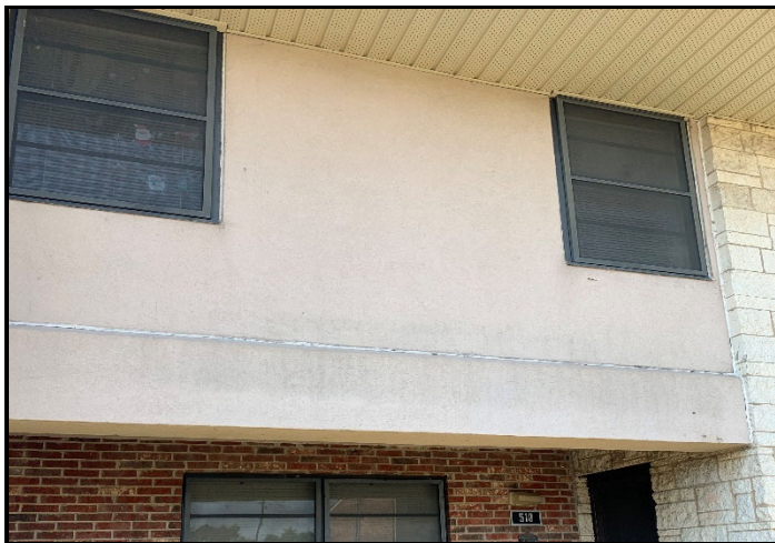
Photo 1: EIFS over former wood batten siding. Poor installation of a faulty produce (CSPC recall on EIFS)
