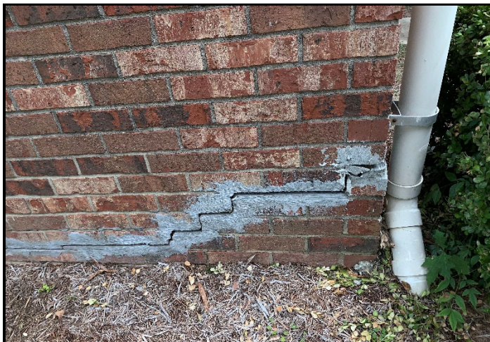
Photo 3: Typical stair step cracking in corners of buildings
