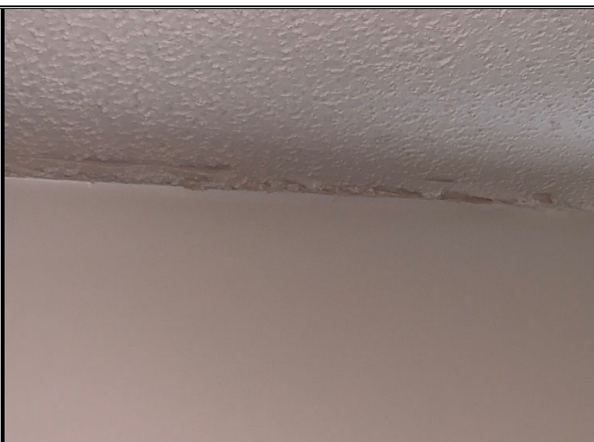
Photo 10: example of structural displacement damage on plaster ceilings and walls of select units
